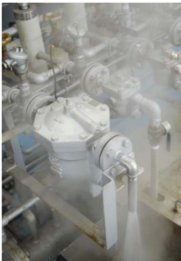
FIGURE 1. Effective steam traps keep heat in the system to optimize production rates and heat quality, and they also discharge condensate to provide for system safety and reliability. Major problems can occur if condensate is not readily drained from the system
