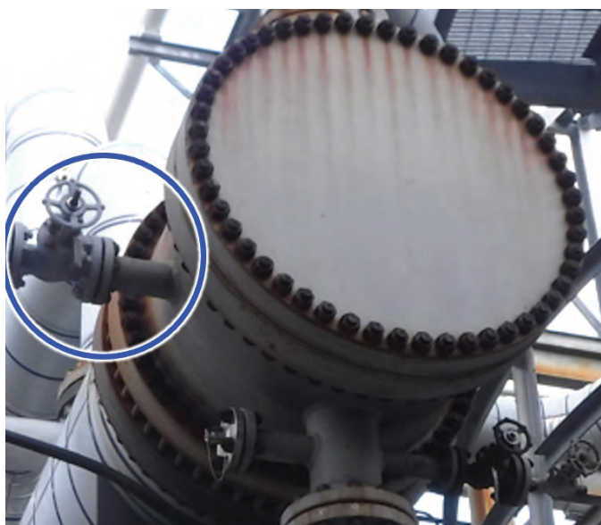
FIG. 11. Tube-side steam reboilers require an outlet-side, channel head large tapping for effective pump/trap operation.
