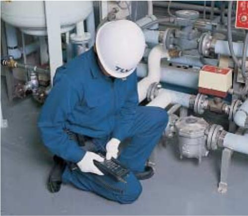
The data required for steam trap management – trap type, size, type of connection, operating pressure, operating status, etc. – can be created and stored in the management log.
